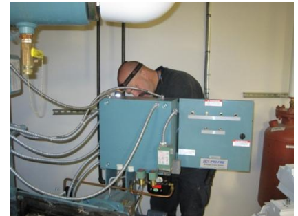
Figure 7 - building automation control work
