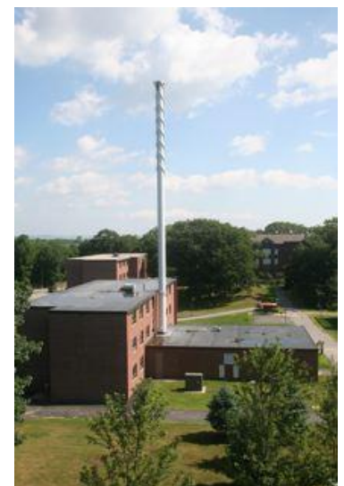
Figure 1 - central heating plant on Biddeford Campus
